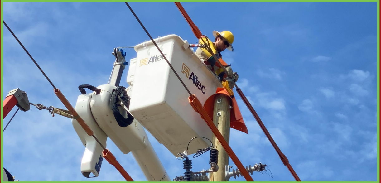
Lineman upgrading infrastructure
